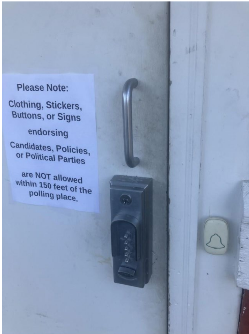
Entrance door to Warwick Town Hall. On the right side of the door there is a vertical door handle. The surveyor noted that the door handle was too high to be accessible.
