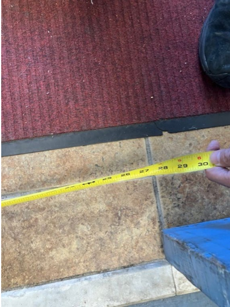
The front entry to the Salvation Army is being measured. The clear space between the doorway measures about 27 inches.
