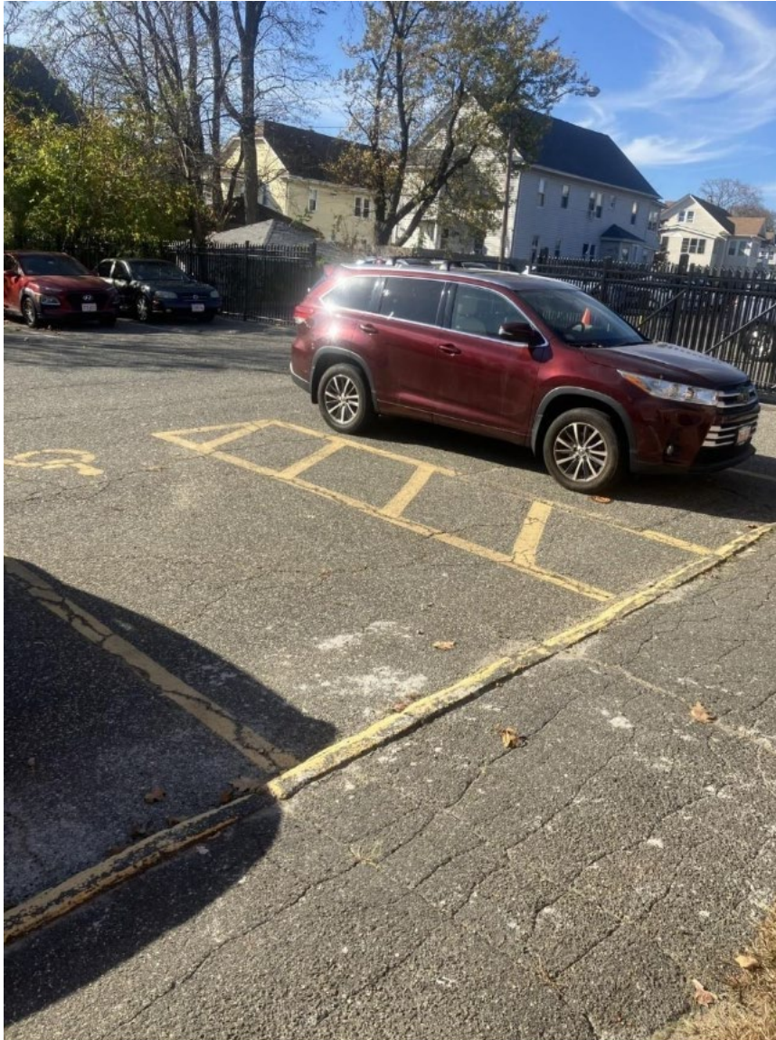
A side view of the accessible parking spaces located directly in front of the Springfield Boys and Girls club polling place entrance. The accessible parking spaces have a curb directly in front of the parking spaces, with no curb cuts.
