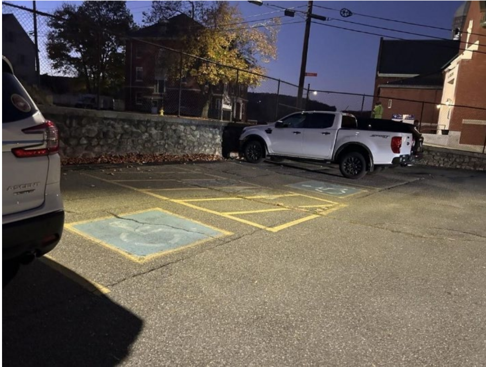
Two accessible parking spaces across the street from Saint Joseph's Catholic Church. The parking spaces have a stone wall directly in front of them and lack a curb cut to the sidewalk.
