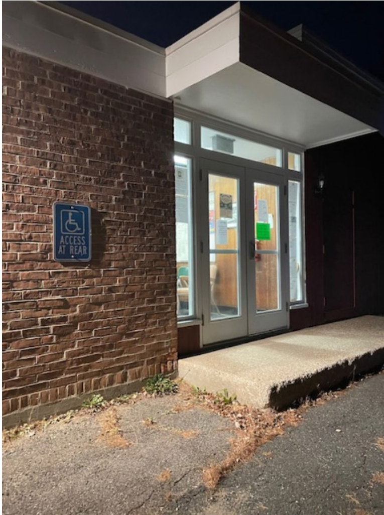
Main entrance to the Washington Town Hall in the evening. There is a blue sign with the international symbol of accessibility reading Access at Rear. There is a cement step and landing leading to the entrance doors.
