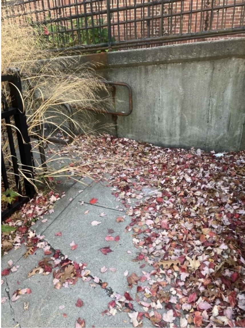
The bottom landing of the ramp at the North End Youth Center. The landing has a thick layer of leaves at the bottom which may be difficult for wheelchair users to navigate over.
