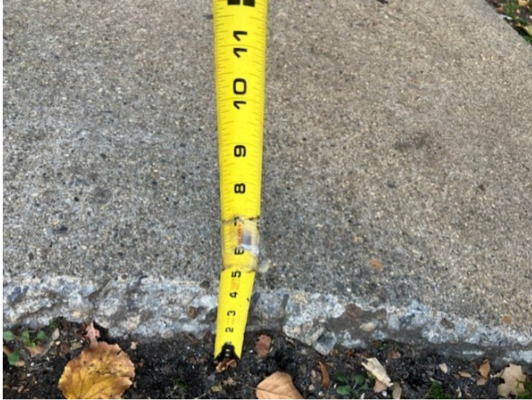
A cement landing with a measuring tape in front of it, showing that the step measures four to five inches.
